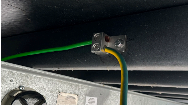
Figure 41 Exterior Grounding Block
