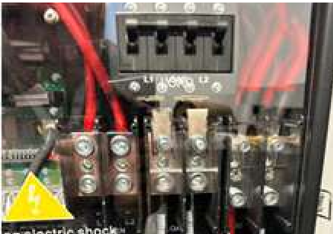
Figure 37 Outgoing Load Breaker Inside of the Inverter
