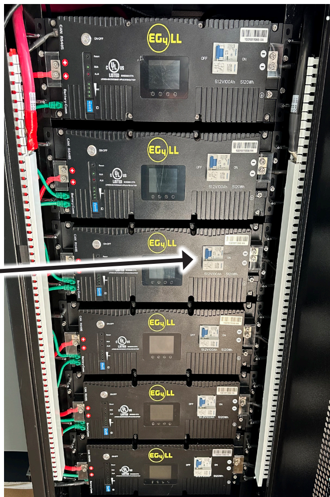
Figure 24 Main Battery Disconnects
