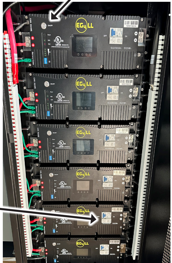
Figure 40 Main Battery Disconnects
