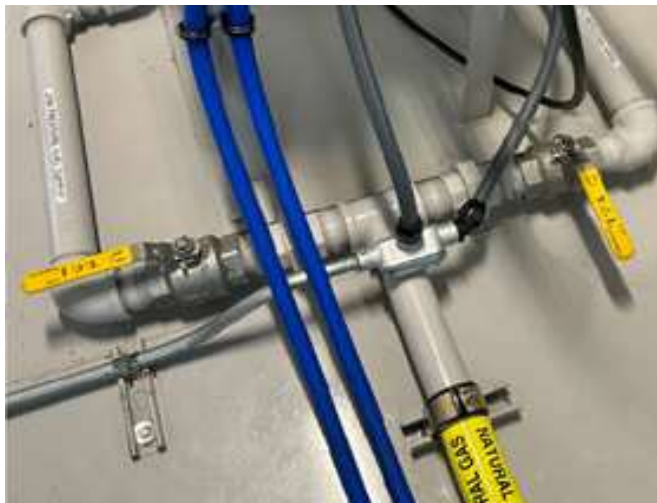
Figure 14 Fuel Source Supply Valves
