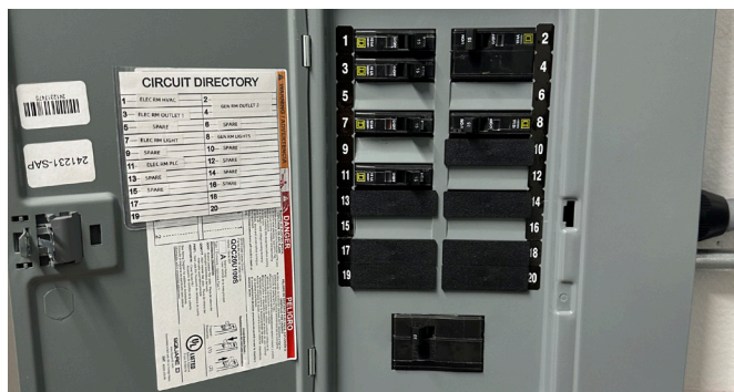
Figure 25 Main Load Center Circuit Breaker
