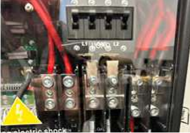
Figure 29 Outgoing Load Breaker Inside of the Inverter
