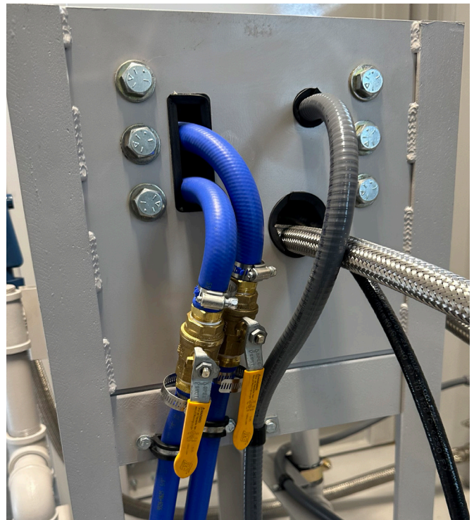
Figure 15 FMM Coolant Valves
