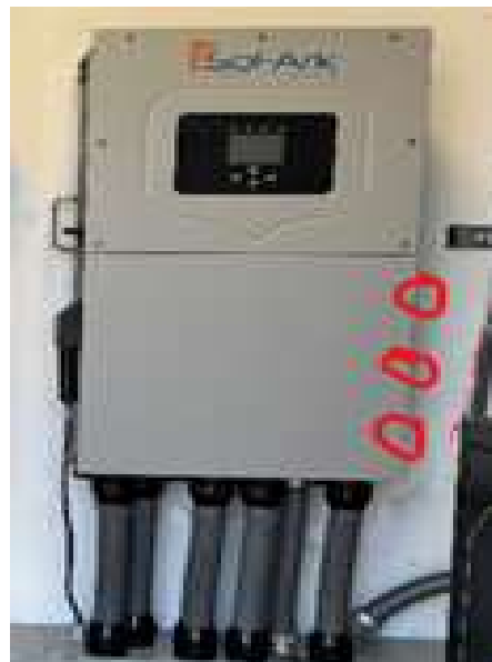
Figure 35 SolArk Inverter
