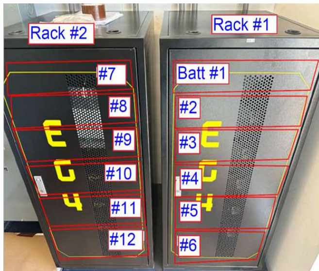
Figure 39 EG4 Battery Rack
